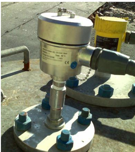
Model SMS2000 Flexible Transmitter Single Cavity Housing
